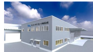
Suzuka Factory, Denko Techno Heat Co., Ltd.
