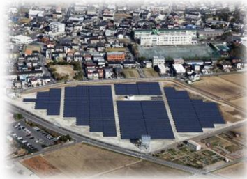
Yosami Solar Photovoltaic Site
