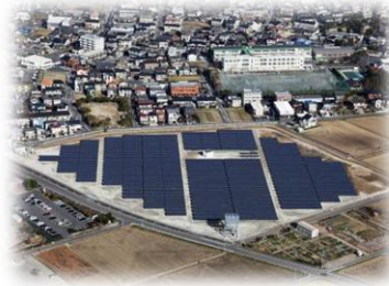
Yosami Solar Photovoltaic Site
